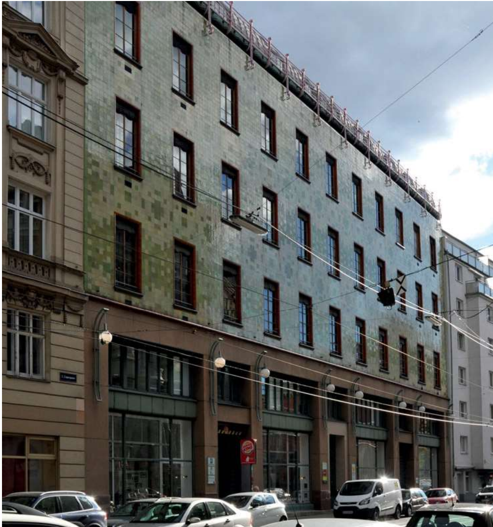
8.26 Portois & Fix apartment and commercial building in Vienna. Max Fabiani, 1899/1900.
