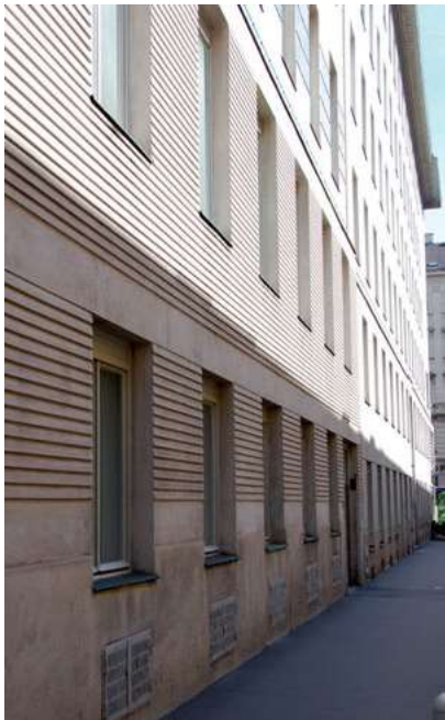
8.20 Granite dressing to the base of the Postal Savings Bank in Vienna. Otto Wagner, 1903–1906.
