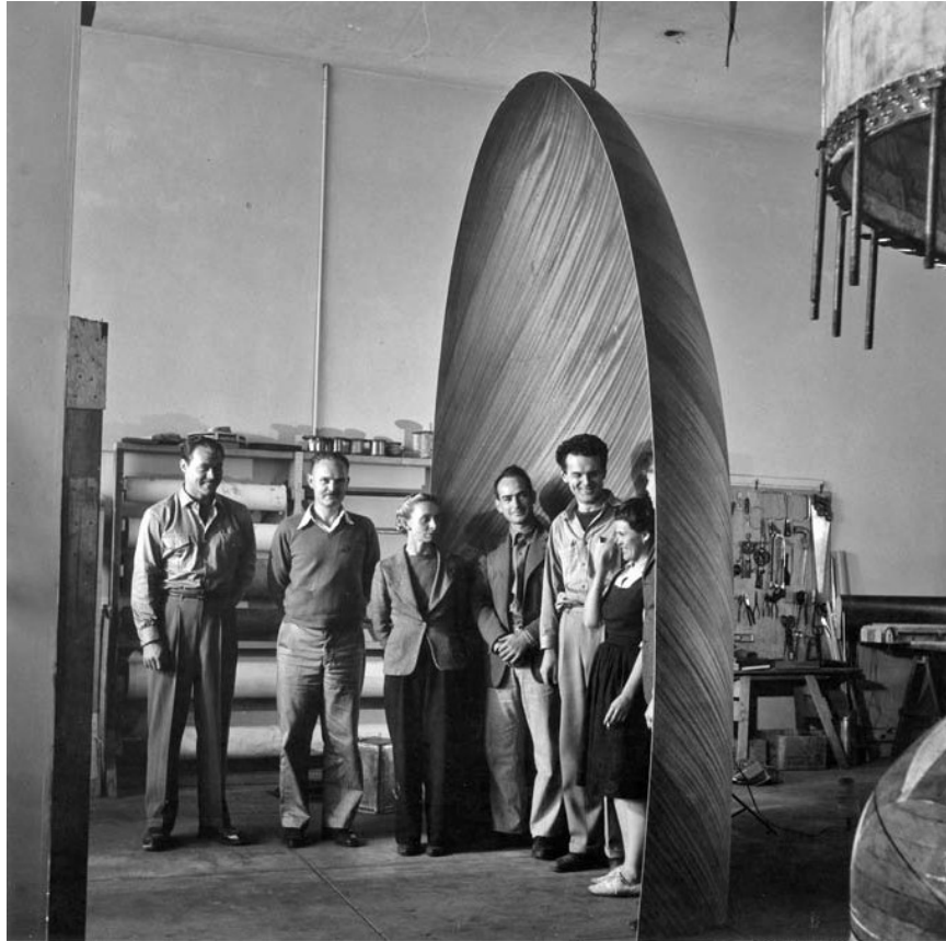
FIGURE 8.2. Molded Plywood Division staff members with a blister for a glider nose section. © 2017 Eames Office LLC (eamesoffice.com).
