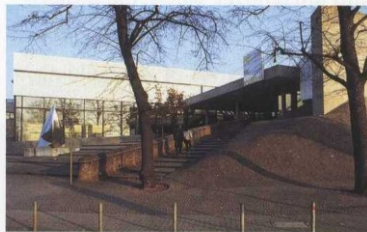
90 Hanover, Sprengel Museum, entrance side
