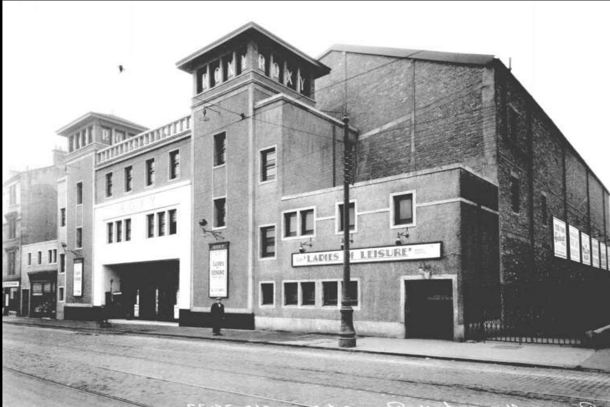
průčelí kina Seamore na Maryhill Road, Glasgow
