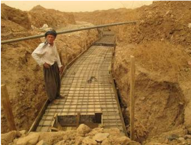
Figure 12. Doundar karez under refurbishment by the KRG Ministry of Agriculture in July 2009. (Photo by Dale Lightfoot)
