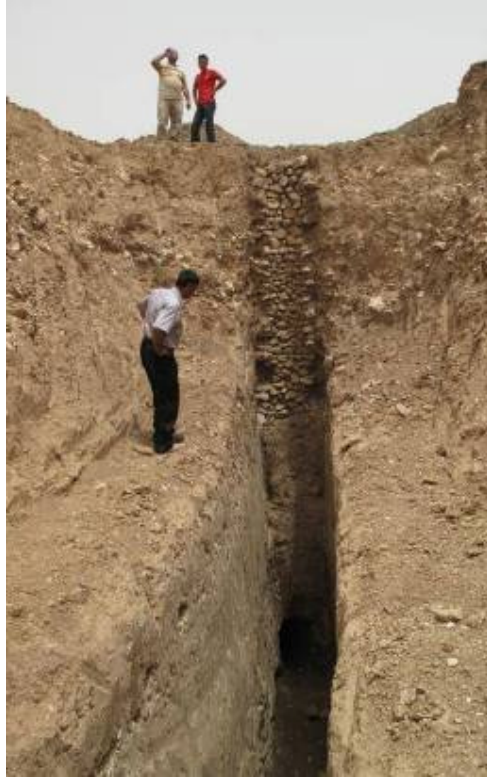
Figure 13(A): Lower section of Barzawan Saru karez at Sewsenan, excavated by Irrigation and Surface Water Directorate of Sulaymaniyah. The upper section of this karez was refurbished the traditional way using wastas who cleaned and reinforced the wells and tunnel (completed July 2009).
