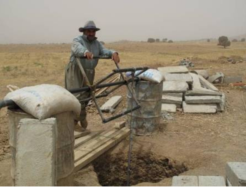
Figure 4. Working a windlass over the mother well of karez Barzawan Saru at Sewsenan. (Photo by Dale Lightfoot)
