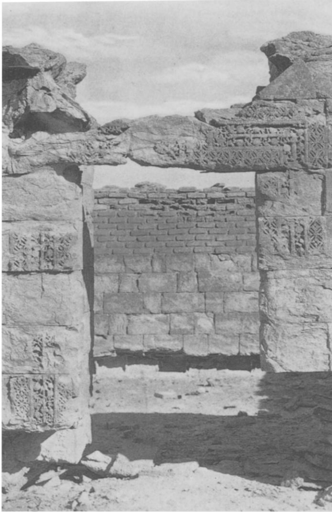
◁ Exterior view of one of the ornately decorated doors in the early eighth-century palace of Qaṣr al-Tuba in the eastern desert of Jordan. Construction of the palace was started but never completed by the Caliph Walid II. The use of brick for the vaulting, visible in the background, is unusual. While explorers documented the site in the 1920s, it awaits further study. From Jaussen and Savignac 1922:pl. 11.
