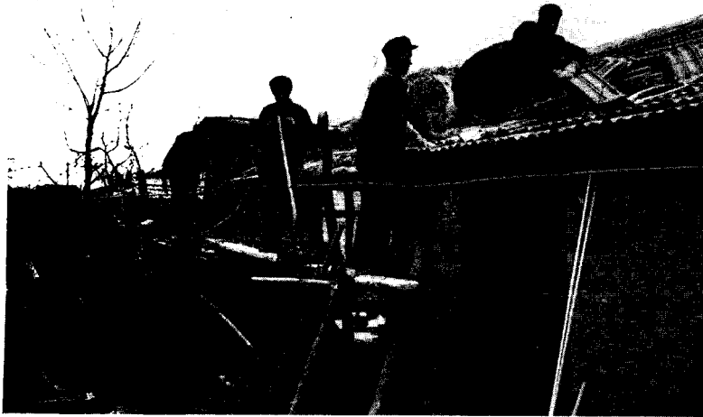
Figure 6 Neighbors assisting with house construction.
