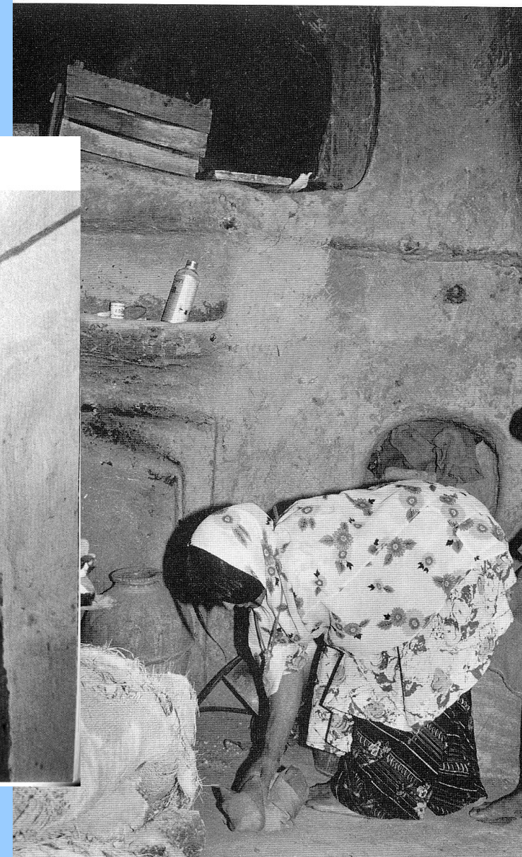
Figure 12. Qal'a Baghestan interior. This abandoned living room has a carved and painted fireplace wall. The plaster on the lower part of the walls was polished with a stone until it shone like marble.
