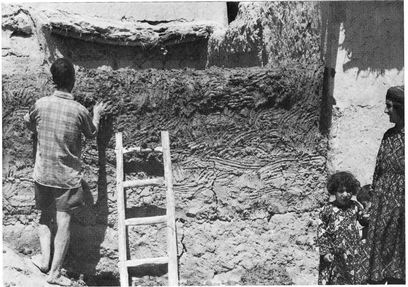
Figure 4.4. Wall construction (packed mud and mud plaster), Aliabad.
