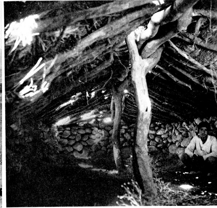
Fig. 8.—Zemgā. Room for live-stock. A low manger to the left. The forked posts carry 1-3 parallel ridge-poles. The rafters are laid between the ridge-poles and the walls. Malāk Hasan to the right. 17. IX. 1964.
