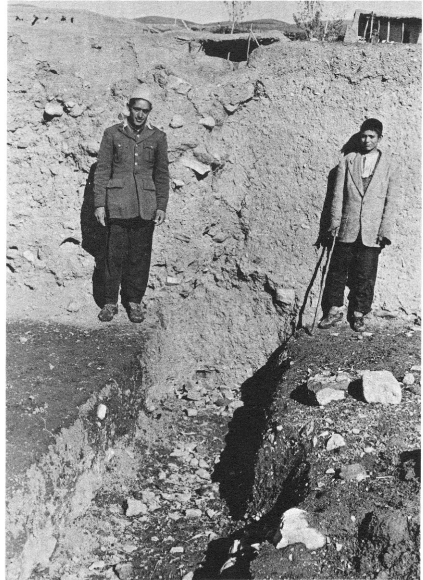
Pl. 5.1. Hasanabad. Footing trench for mud wall. Trench is 90 cm wide and 60 cm deep.
