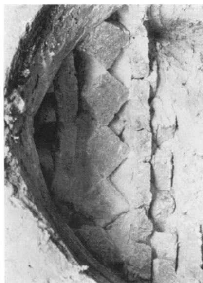
FIG. 23.—Brick decoration in room 17.
