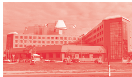
The new building of the National Archives and central Bohemia's Regional State Archives in Chodovce, Prague.
