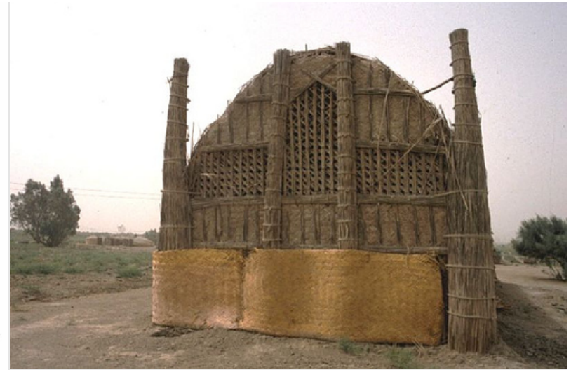
Reed houses ( mudhif ) are built up to the present day in the marshes of Iraq Southern Iraq
