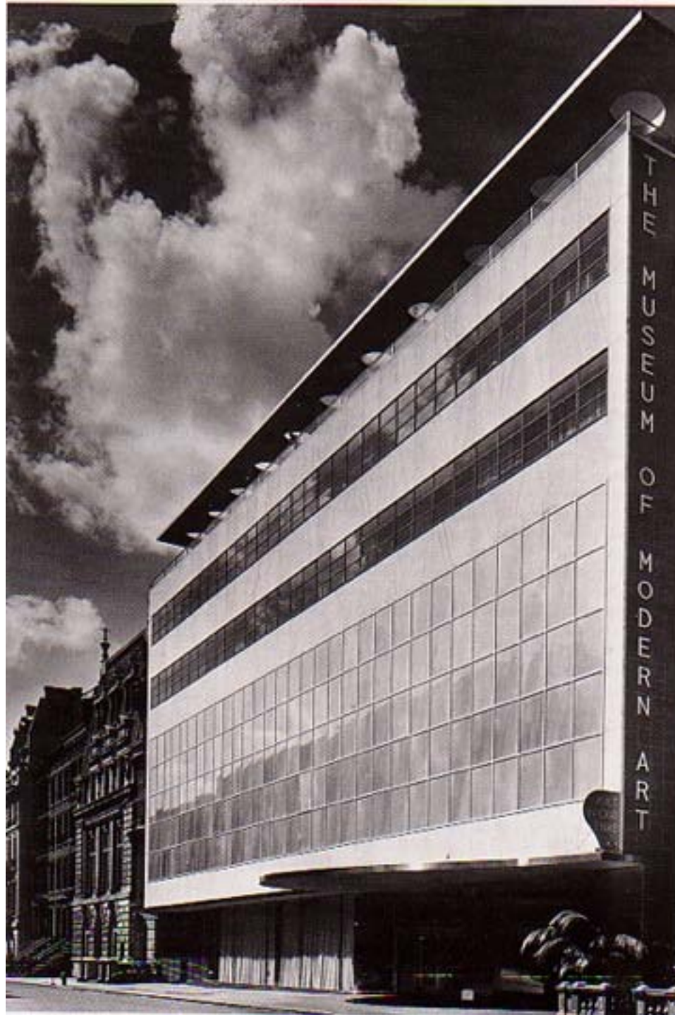
MOMA, designed by Philip L. Goodwin & Edward D. Stone, 1939
