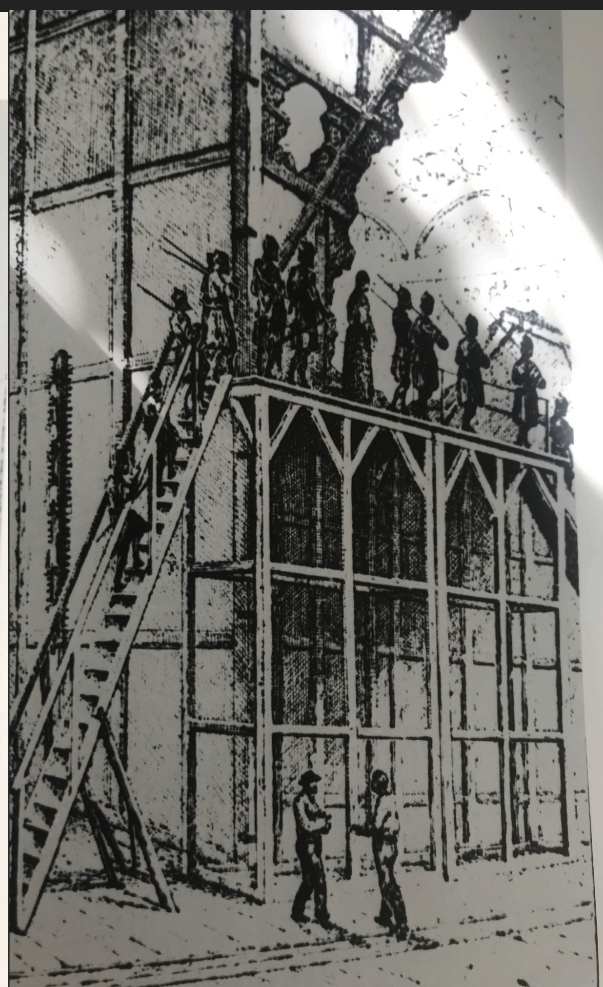
FIGURE 1.21 Isometric drawing of stage right showing the masonry proscenium wall, wooden bridges, stage floor slots, and scenery. [Yale Print Collection.]
