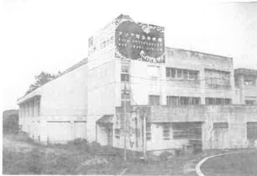
TOP: Aerial view of 3331 Arts Chiyoda, converted Renzei Junior High School, near Akihabara. Courtesy of 3331 Arts Chiyoda. BOTTOM: Asia Photography and Image Center, former Miyokoyama Primary School, Echigo-Tsumari (2012). Photo by author.
