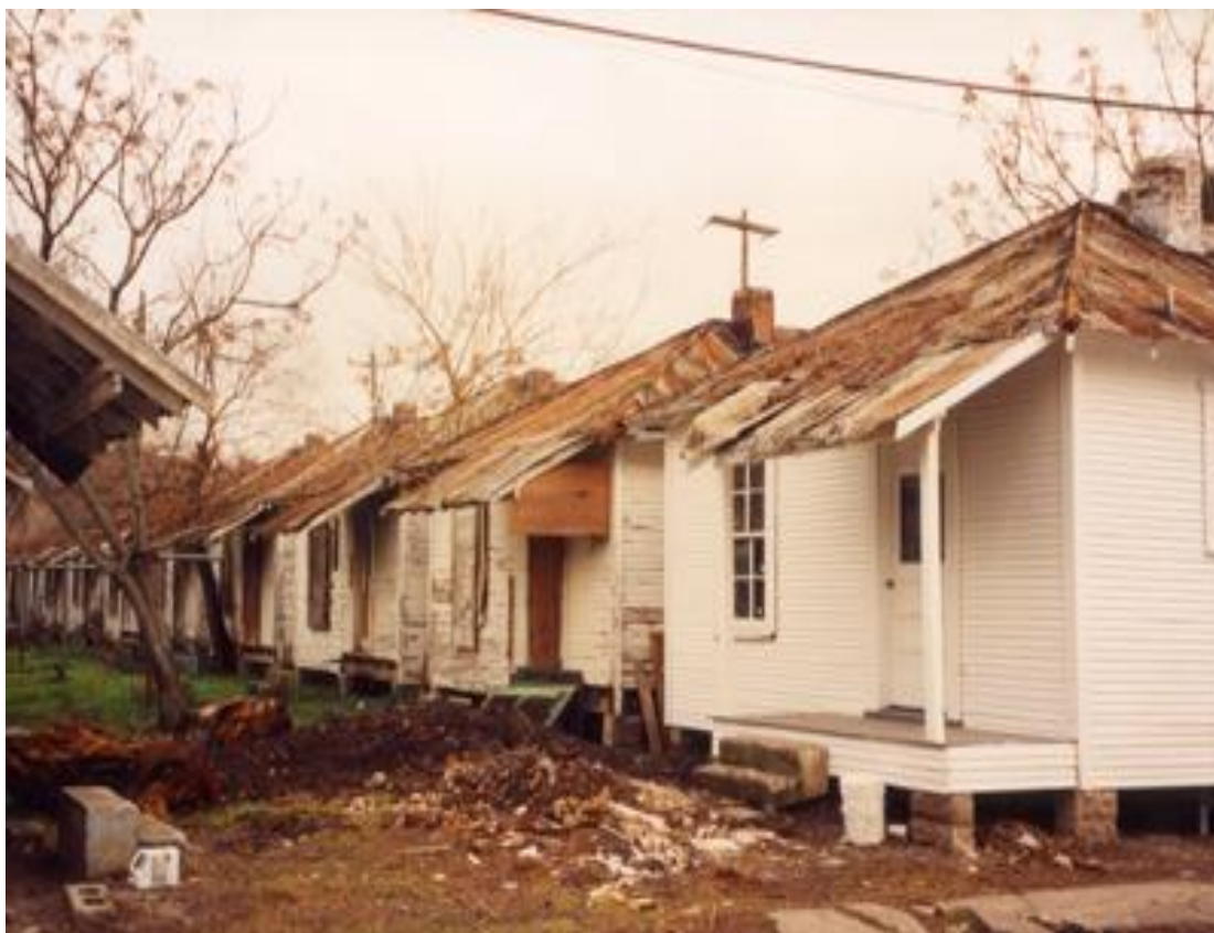
[Fig. 8] Photograph of PRH before renovation. January 1993. Courtesy of PRH
