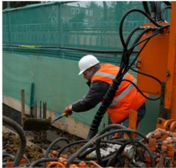
construction worker in orange safety vest is working on road.
