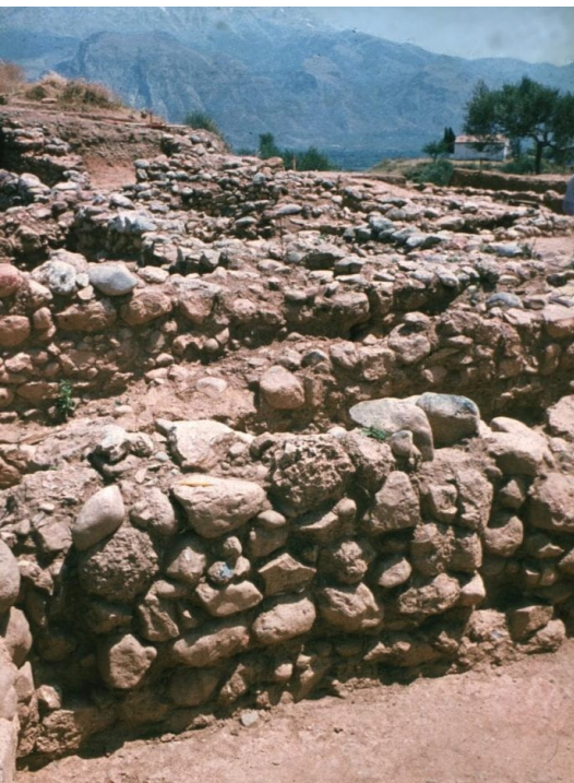
Menelaion. Period I Mansion (LH IIB): Rubble Wall with Vertical and Horizontal Beam Slots.
