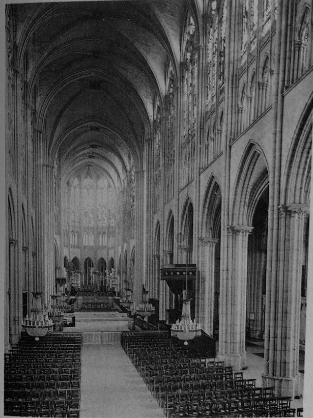
Figure 22. St.-Denis, interior of the nave. Begun 1231.
