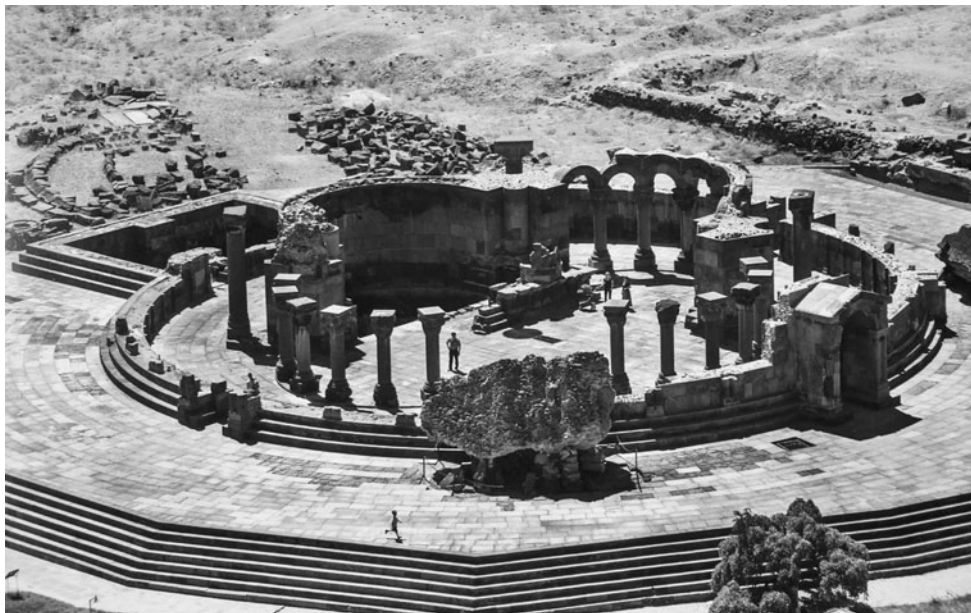
Figure 2.5 Church of Zuart'noc', Republic of Armenia, ca. 641–ca. 661, aerial view. Photograph courtesy of Hrair Hawk Khatcherian.
