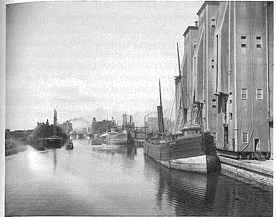
Unloading grain at the Great Northern Railroad elevator in Buffalo, New York, ca. 1900. Given the enormous amounts of grain on the move, methods of storing, cleaning, drying, and transferring the grain became indispensable. Major flour corporations built multiple manufacturing plants closer to the sources of production and sought out sites that reduced their transaction costs. Thanks to the rise in importance of the Great Lakes as a conduit for western US and Canadian wheat, and the abundance of cheap electrical power from Niagara Falls, by 1930 Buffalo was the world's leading milling center. (Library of Congress)
