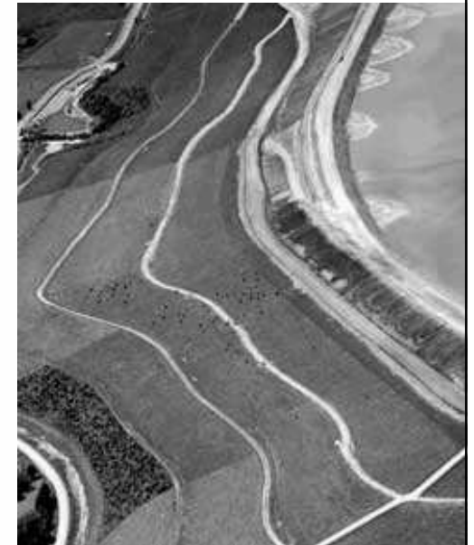
Above: Tailings Storage Facility 2 showing the tailings beach and rehabilitated slopes of the waste rock embankment.
