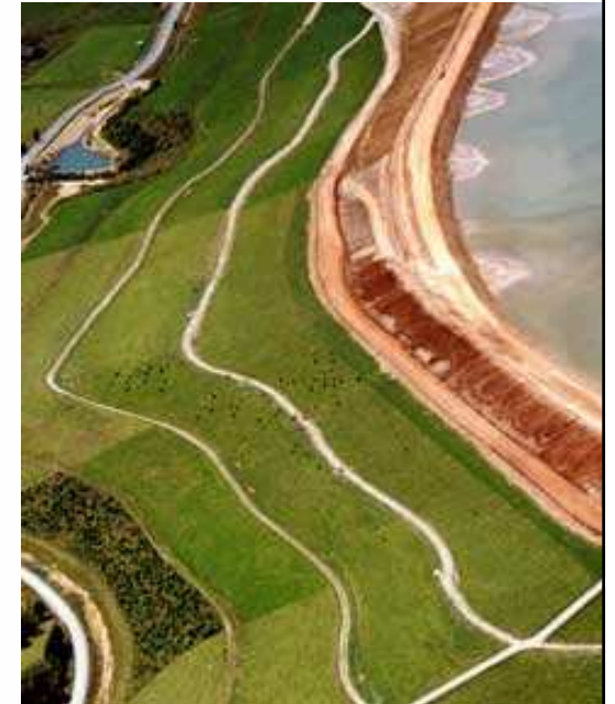
Above: Tailings Storage Facility 2 showing the tailings beach and rehabilitated slopes of the waste rock embankment.
