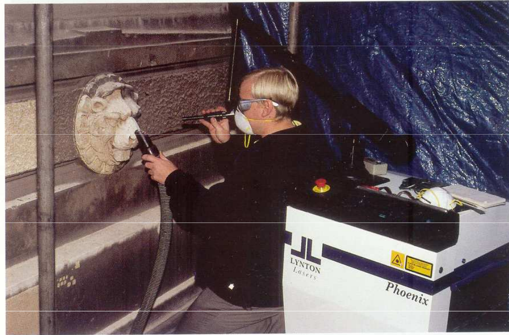
Plate 4.1. Laser cleaning of sculptural detail on the outside of a building.
