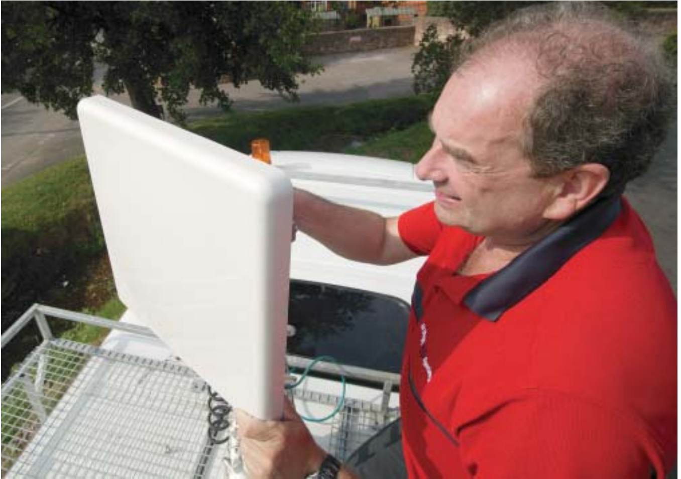
Broadband installation, Buckfastleigh broadband project, Devon
