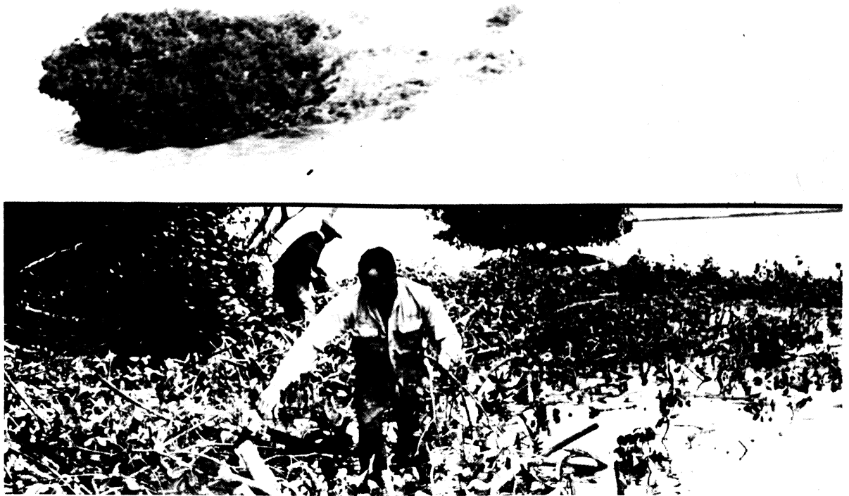
FIG. 5. Upper : Island R1 as tide comes in when removal of right-hand section is nearly complete. Lower : Removal of roots on island R1; process was continued until water covered tops. Note satellite island in background.
