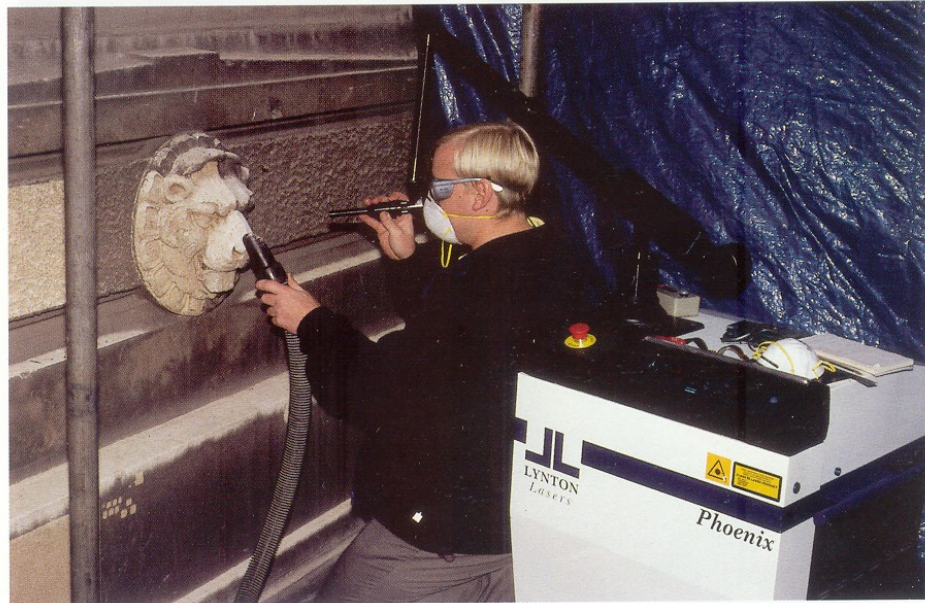
Plate 4.1. Laser cleaning of sculptural detail on the outside of a building.
