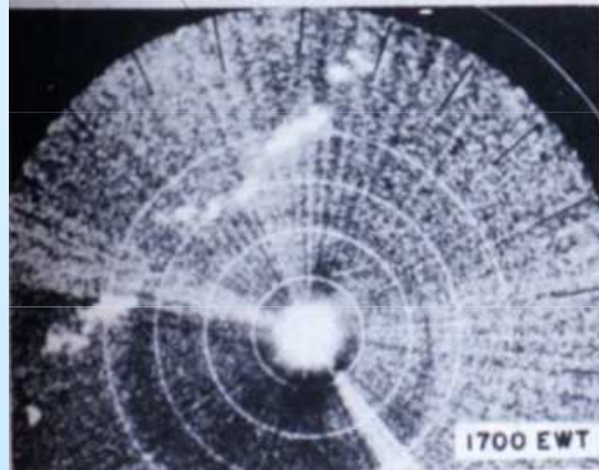
Figure 74. Approach of Cold Front Detected by X-Band Set, 22 July 1943, Boston, Mass. Range markers are at 20-mile intervals. Storms associated with front show considerable motion during the interval between 1630 and 1645 EWT, but very little motion thereafter.
