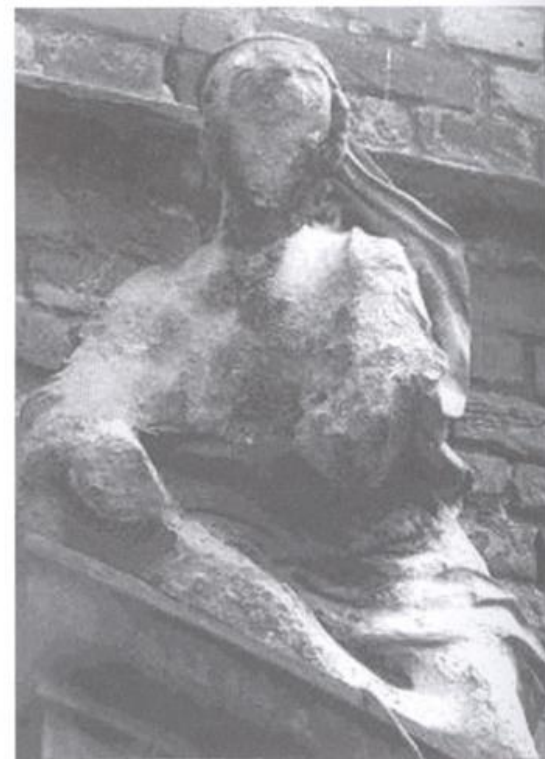
Figure 10.6. Sandstone figure over the portal of a castle, built in 1702, in Westphalia, Germany, photographed in 1908 (left) and in 1968 (right). The erosion of the figure is due to a combination of acid deposition and air pollution produced from the industrialized Ruhr region of Germany. Courtesy Herr Schmidt-Thomsen.
