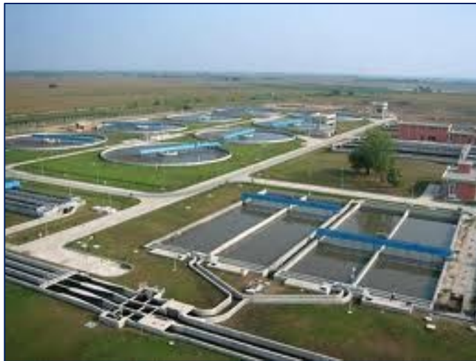
WWTP – Waste Water Treatment Plant
