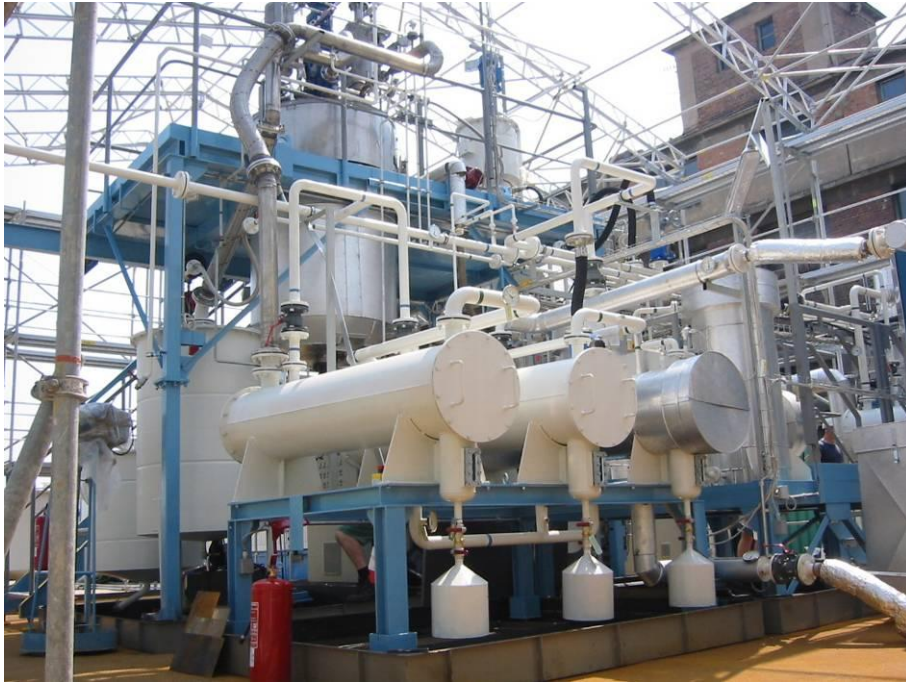
Pilot Plant Erection, Spolana
