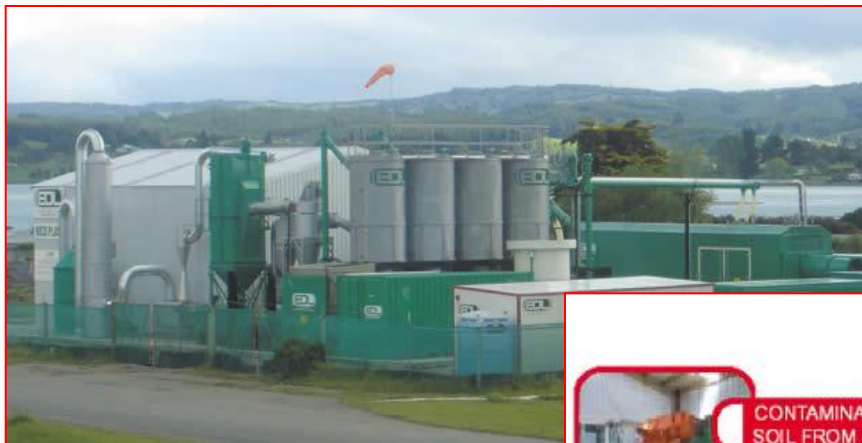
Full scale EDL's MCD plant in New Zealand
