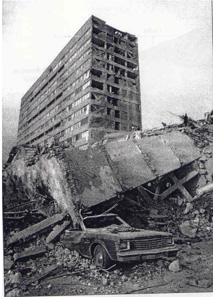
FIGURE 10.9 Mexico: earthquake damage. Some buildings collapsed during the 1985 earthquake in Mexico City, causing loss of life and property. Others remained standing but suffered some damage.
