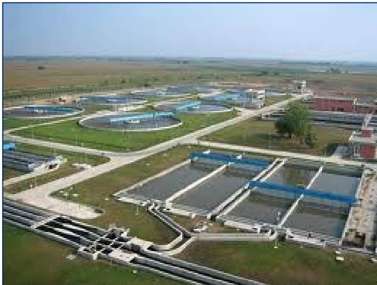
WWTP – Waste Water Treatment Plant
