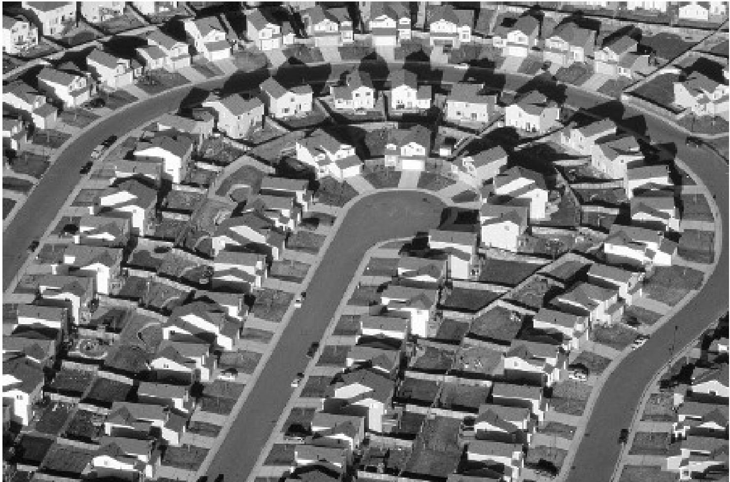
■ FIGURE 1-2 Sprawl on a neighborhood scale. This configuration is sometimes called “loop and lollipop” development. Note the monotonous architecture, the exclusively residential land use, poor connectivity, and automobile dependence.
