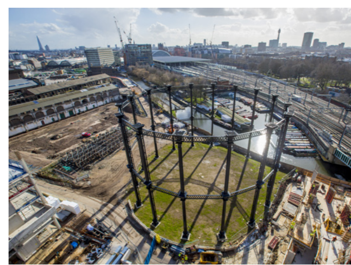
The refurbished and rebuilt Gasholder No.8 forming Gasholder Park © John Sturrock
