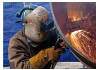
Construction on site © John Sturrock
