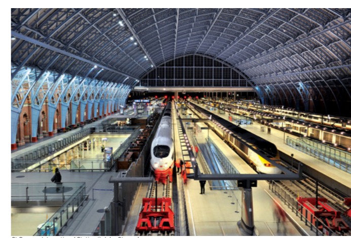
St Pancras International Station © John Sturrock
