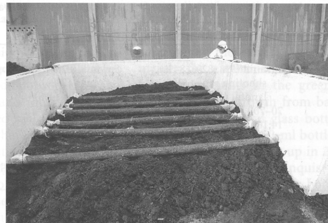
Fig. 22.5. Pilot pile for the treatment of contaminated sawmill soil by the fungal tube technology. The pile works with a volume of 12 \text{ m}^3 ( 3 \times 4 \times 1 \text{ m} ) and finally contains 7 t of contaminated soil. Six fungal tubes are still visible, but are later covered with soil as well
