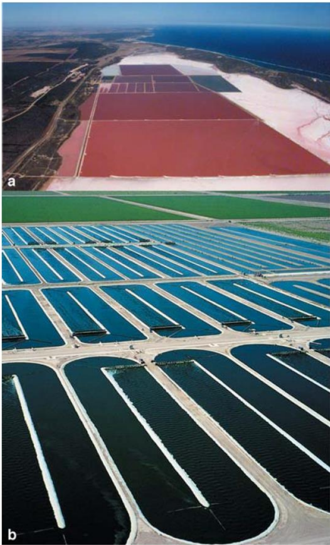
FIGURE 14.1. (a) Extensive open ponds at the Hutt Lagoon, Western Australia, plant operated by Cognis Nutrition & Health, growing D. salina as a source of natural beta-carotene. The largest ponds are about 200 ha in area. (b) Raceway ponds used for the culture of Spirulina by Microbio Inc. at Calipatria, California (photo courtesy of Dr. Ahma Belay).
