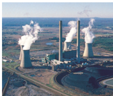
Figure 6-10 Georgia Power Company's Plant Bowen at Taylorsville, Georgia. Plants such as this one burn more than 10^7 tons of coal and produce over 2 \times 10^8 megawatt-hours of electricity each year.
