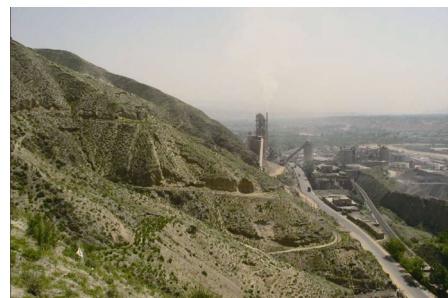
Figure 8 Fault scarp at the boundary between the Laoya block composed of hard rock and the Minhe depression underlain by soft sediments
