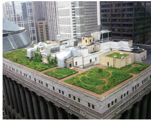
Figure 1: Chicago City Hall Green Roof
