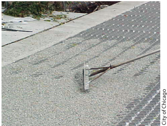
Raking gravel into a Gravelpave2 system.
