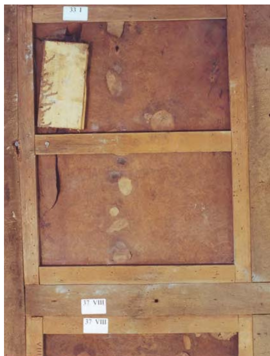
Figure 23.74 Old leather patches on the back and a more recent repair with timber.
