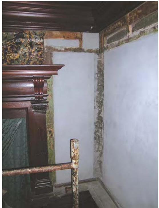
Figure 23.93 Wall after replastering ready for leather to be rehung.
