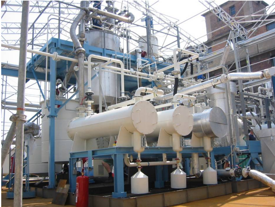
Pilot Plant Erection, Spolana
