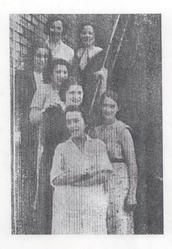
Fig. 1.5. Selenyi's Electrographic Reproduction Image resulting from scanning with his triode in air and powder development. (Reproduced from Wireless Engineer, June 1938, Fig. 4 of article "Application of Electrography in Television," by P. Selenyi. Permission granted to reproduce.)
