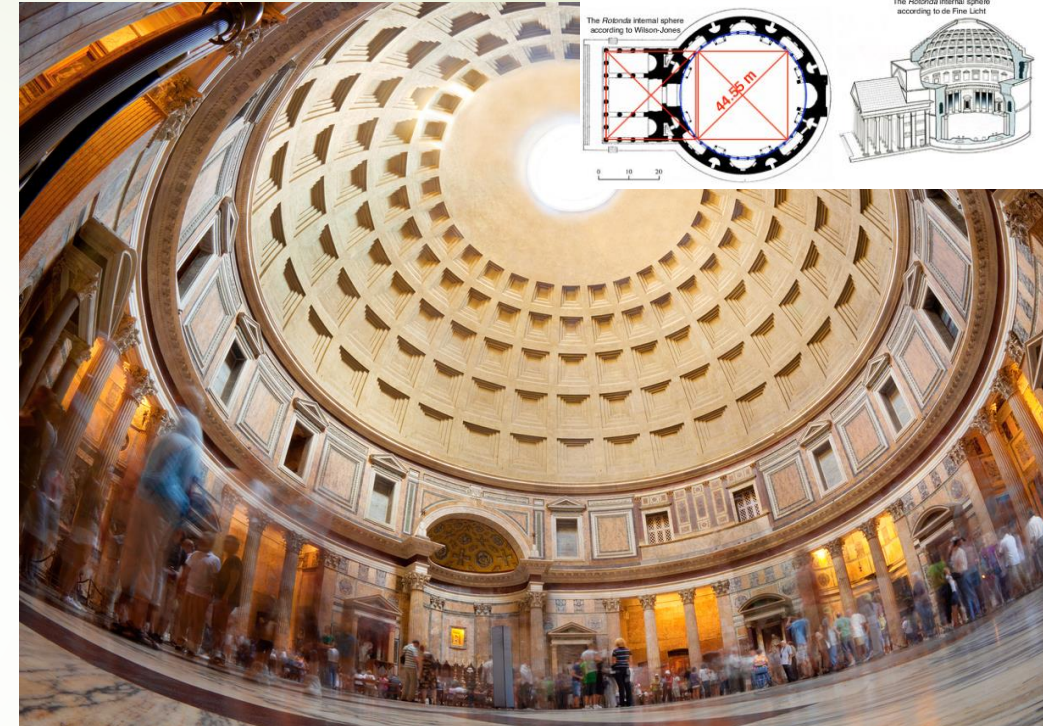
The Pantheon (completed around 126-128 A.D) in Rome features the world's largest unreinforced concrete dome.
