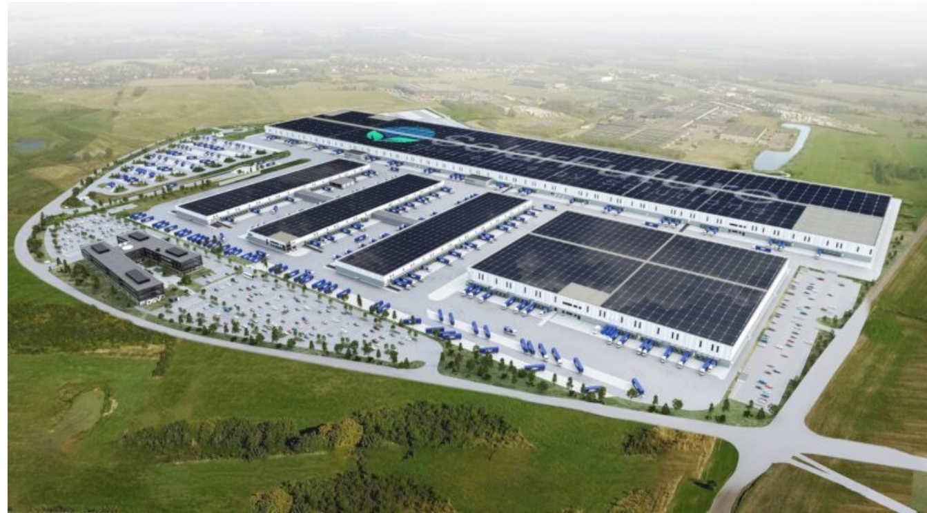
35 MW rooftop solar power plant at DSV's new logistics center in Horsens – to be completed in Dec 2024 (cleantechnica.com)
