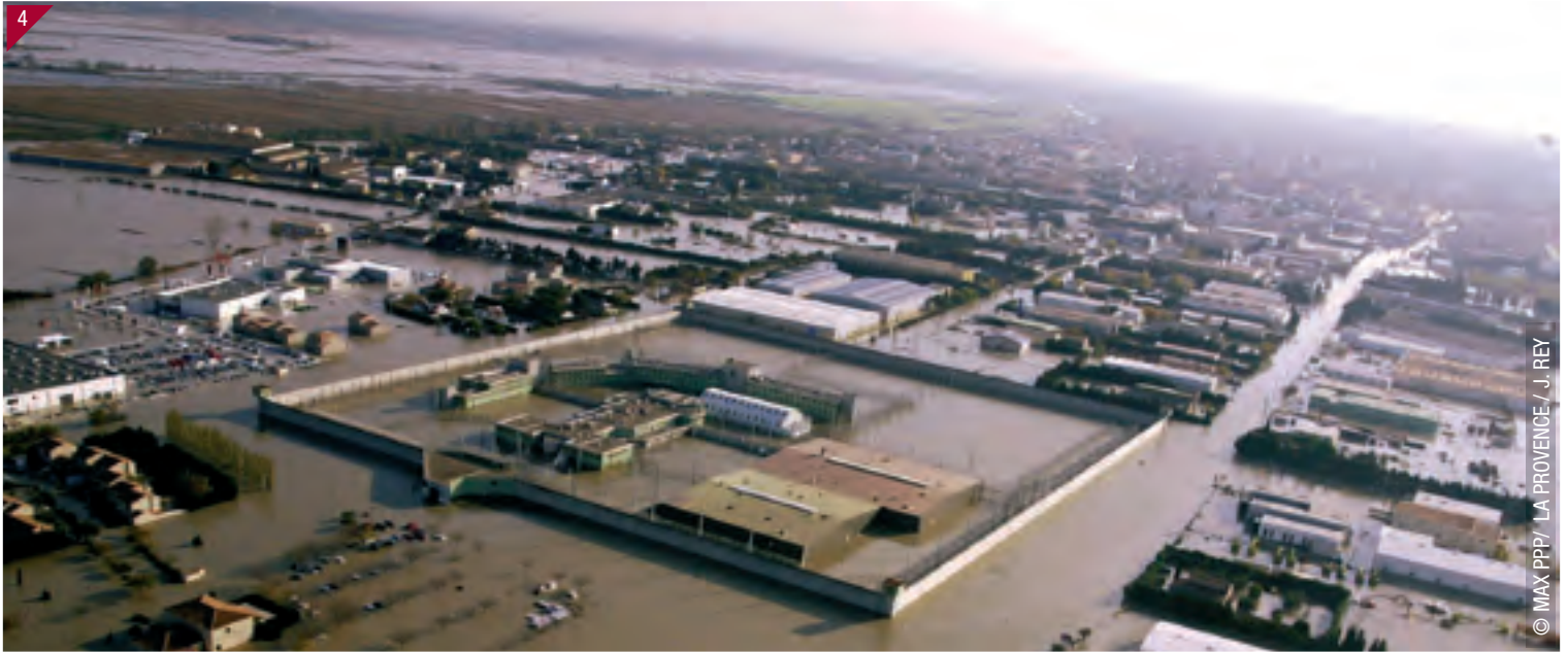
Arles submerged by flooding (7th December 2003). Although the natural phenomenon of such sudden and heavy rainfall is nothing new, infrastructures put in place by humans exacerbate the consequences.
